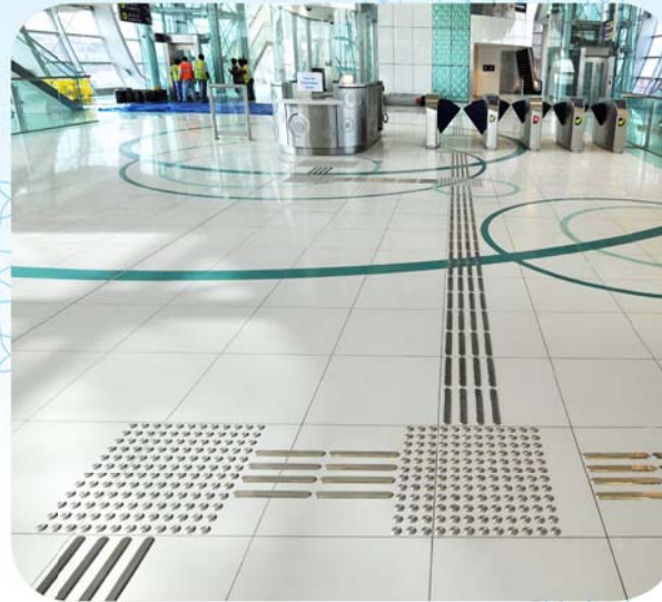
Tactile guidance path in every station.
